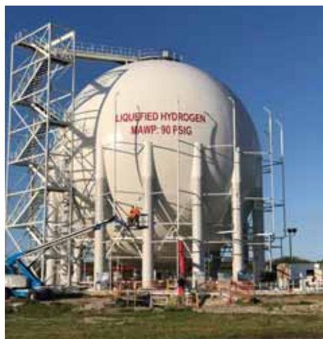
Figure 1. New NASA \text{LH}_2 storage tank during painting. Credit: CB&I
